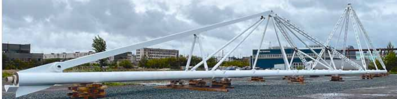
Fig. 5. Installation of the assembled boom at the manufacturer's assembly site
