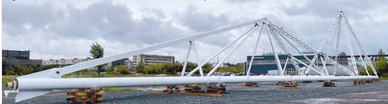
Fig. 5. Installation of the assembled boom at the manufacturer's assembly site
